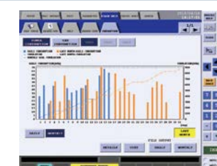
Power consumption monitor
